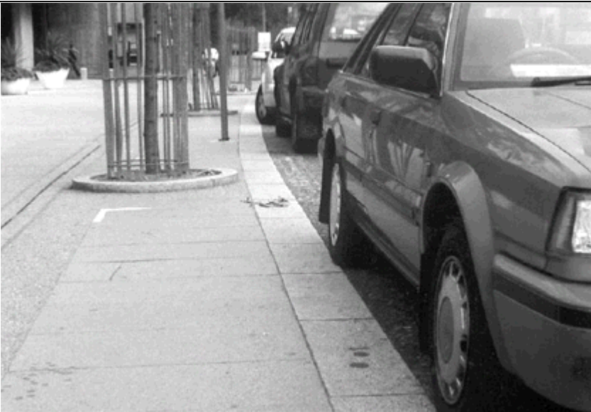
Kerb free level access parking bays with a transfer area defined by surfaces, textures and planting. This avoids the use of painted lines on the road and pavement.
